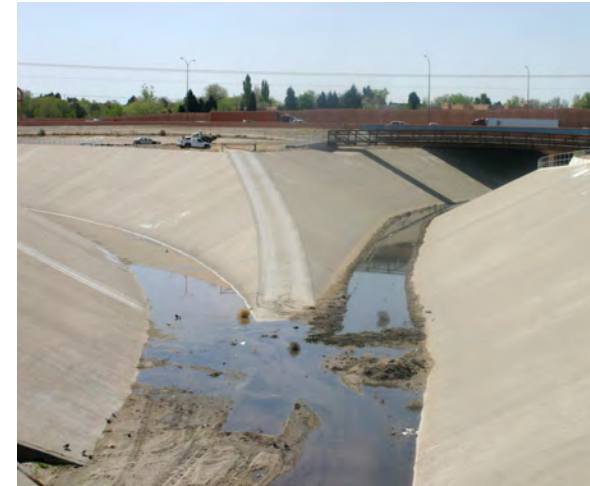
Figure 1 Concrete lined arroyos in Albuquerque, New Mexico
