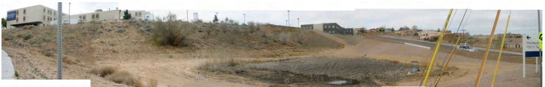
Figure 4 Stormwater detention basin on the Lovelace Hospital West Side campus in Albuquerque, NM
