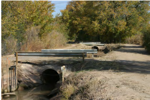
Figure 14 An open water irrigation drain in Albuquerque's North Valley.
