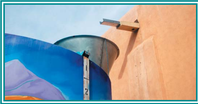
Cistern Collecting Roof Runoff
