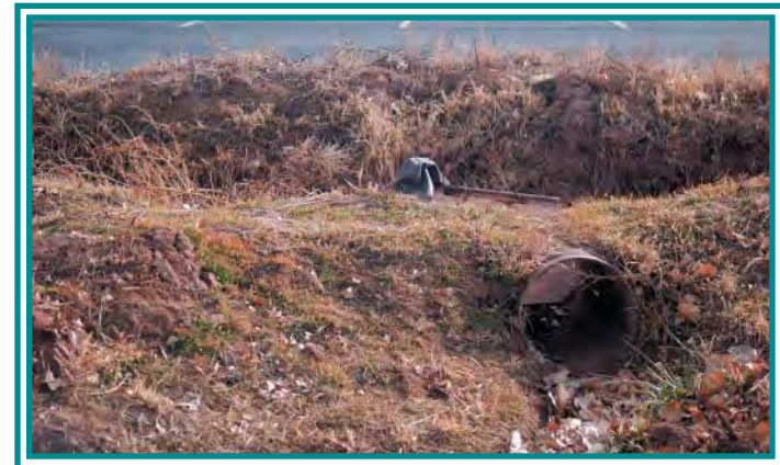
Diverting Irrigation Water From the Ditch
