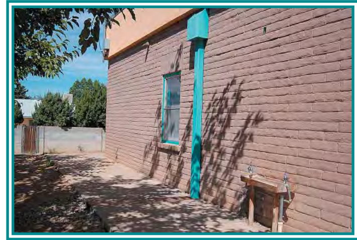
B-Building Roof Drain, North Side
