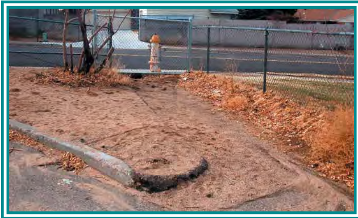
Southwest Corner Drain to Street
