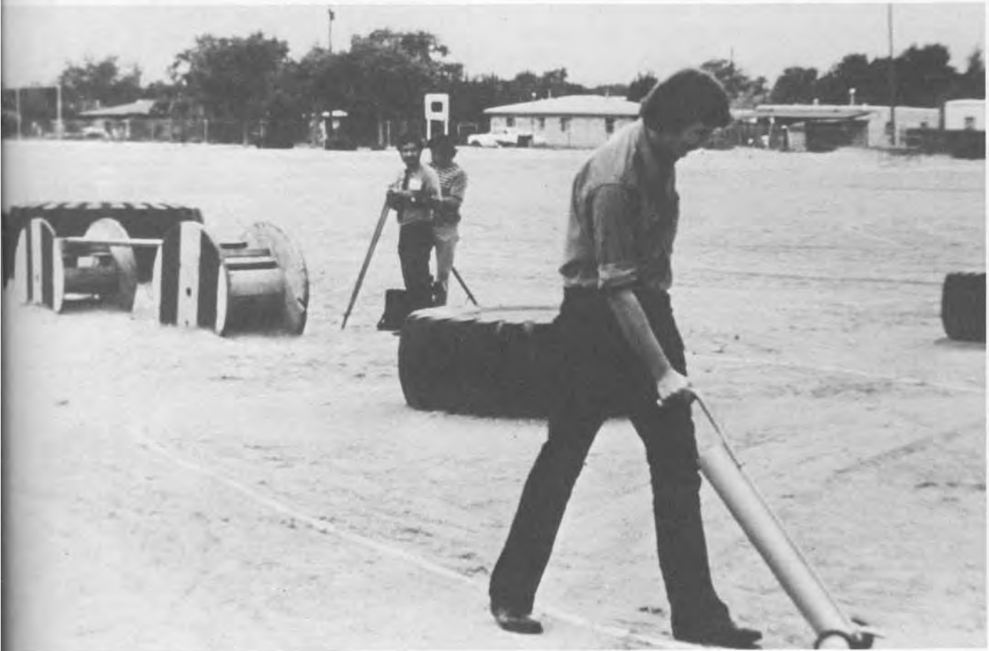
The district maintenance and operations crew take a core sample to determine the water table level.
