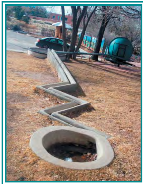
Concrete Channels Collect Water...
