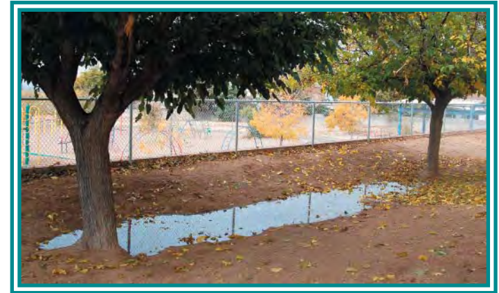
Drainage Collected in the North-South Ditch
