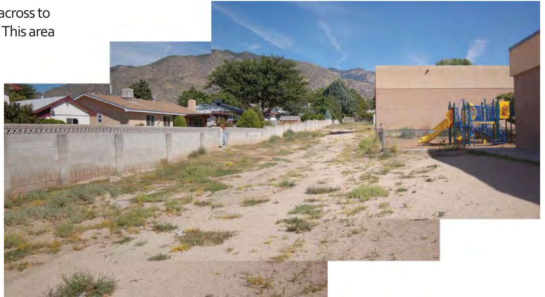
North Side of B-Building: Looking East
