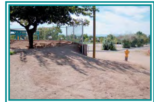
North Side Retaining Wall Termination
