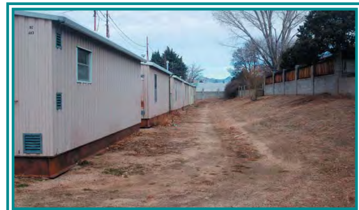
Area Behind Portables: Vehicle Access
