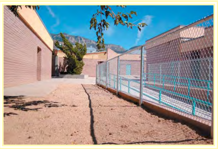
Flat and Narrow Stretch of Soil Between B-Building Front Door and Ramp to Playground
