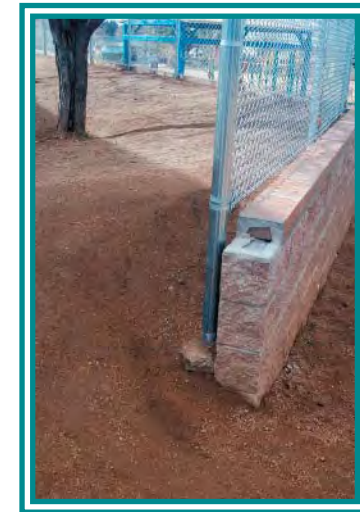
Detail of Exposed Wall Foundation
