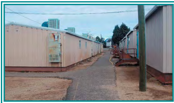
Portable Classrooms: Looking North
