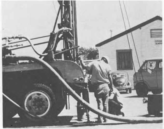
The district maintenance and operations crew take a core sample to determine the water table level.
