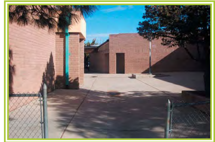
Main Entry Area
