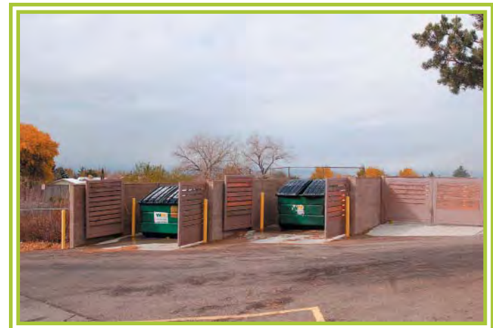
Dumpsters and Entrance to Service Area
