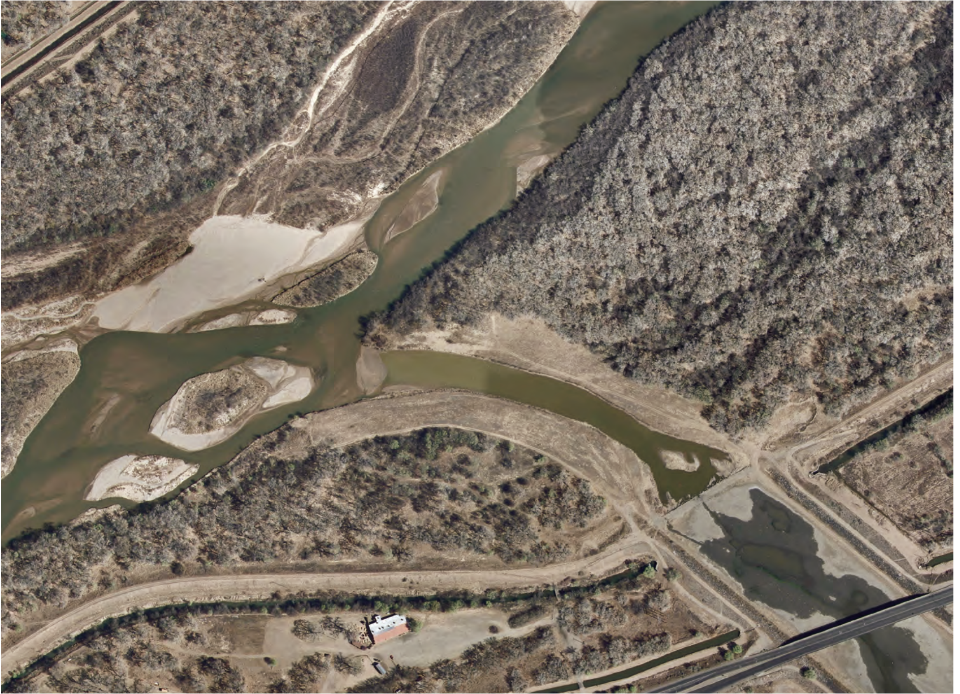
Existing pilot channel conditions. Note: plug at outlet crossing, stagnant water, and low DO problems, as well as the unnatural shape and 'grubbed' area that is devoid of most species that should be present at this site.
