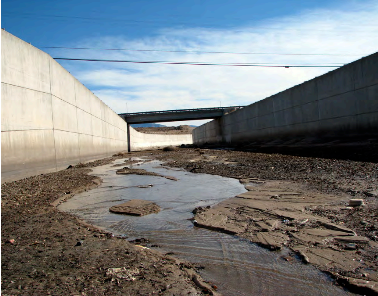
North Diversion Channel
