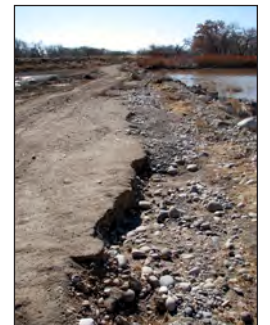
'Equipment crossing' existing conditions
