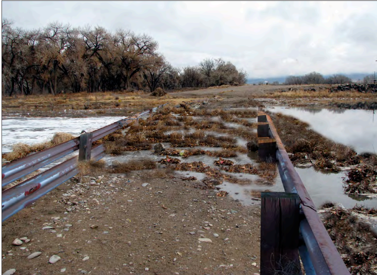
'Equipment crossing' improvements
