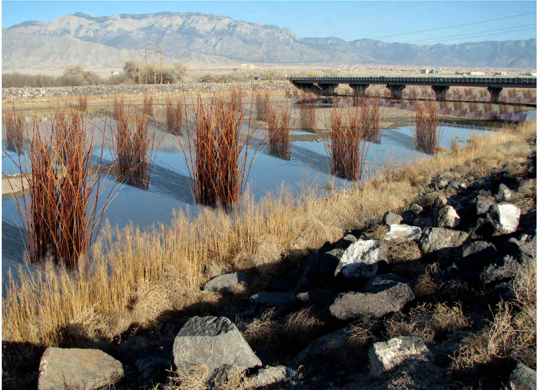
Chevron shaped willow-cart filter islands remove pollutants and create habitat.
