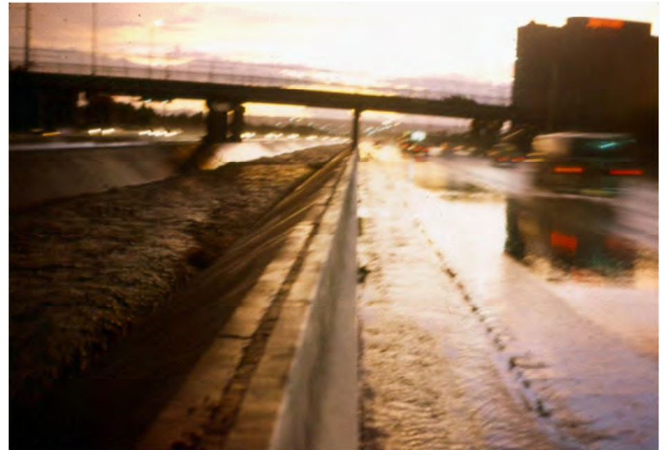
Figure 2. Albuquerque stormwater infrastructure during rain event. Image from amafca.org.
