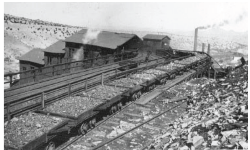
Fig. 23: Historical photograph of the rail lines that ran from mine to mine, from which the gob piles were created.
